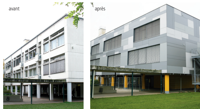
Photos © Rongen Architects
